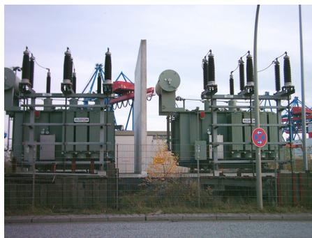
*Power is distributed over large distances at high voltage to reduce power loss in the transmission lines. The voltages generated at the power plant are stepped up by passive devices called transformers (see [Transformers](#)) to 330,000 volts (or more in some places worldwide). At the point of use, the transformers reduce the voltage transmitted for safe residential and commercial use. (Credit: GeorgHH, Wikimedia Commons)*
