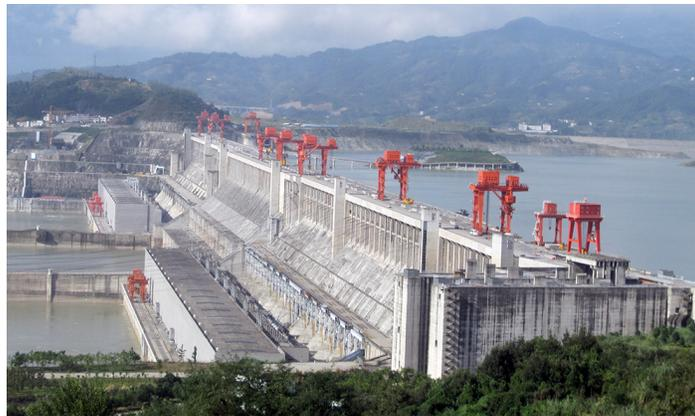
*Three Gorges Dam in central China. When completed in 2008, this became the world's largest hydroelectric plant, generating power equivalent to that generated by 22 average-sized nuclear power plants. The concrete dam is 181 m high and 2.3 km across. The reservoir made by this dam is 660 km long. Over 1 million people were displaced by the creation of the reservoir. (credit: Le Grand Portage)*
